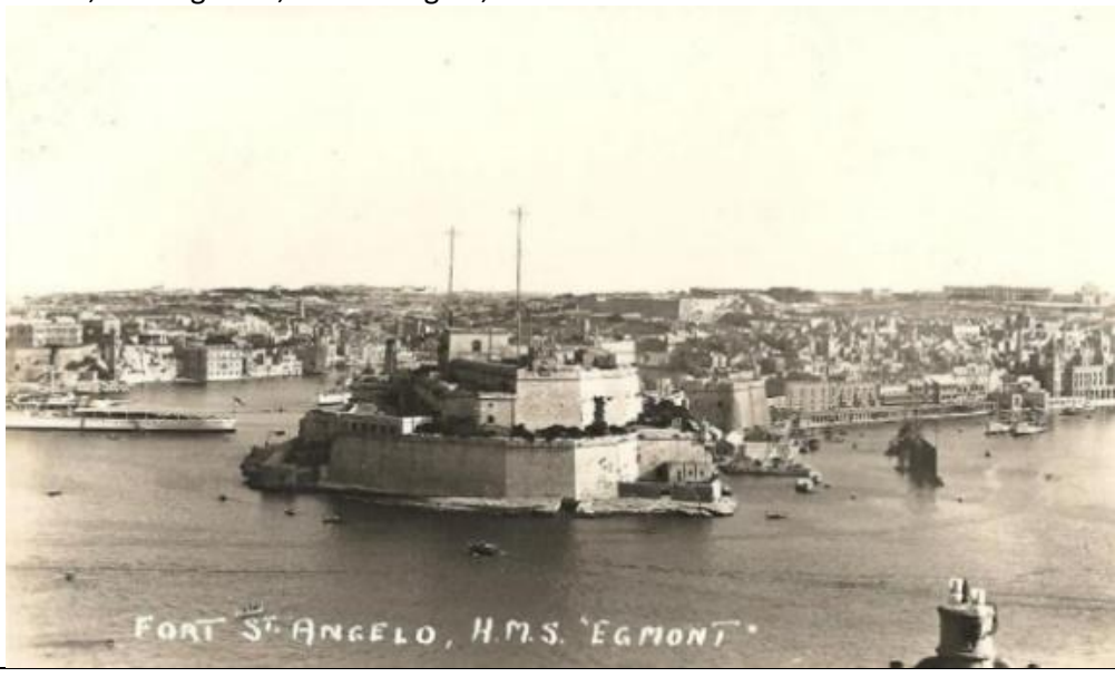
Below, HMS Egmont, Fort St Angelo, Malta.
